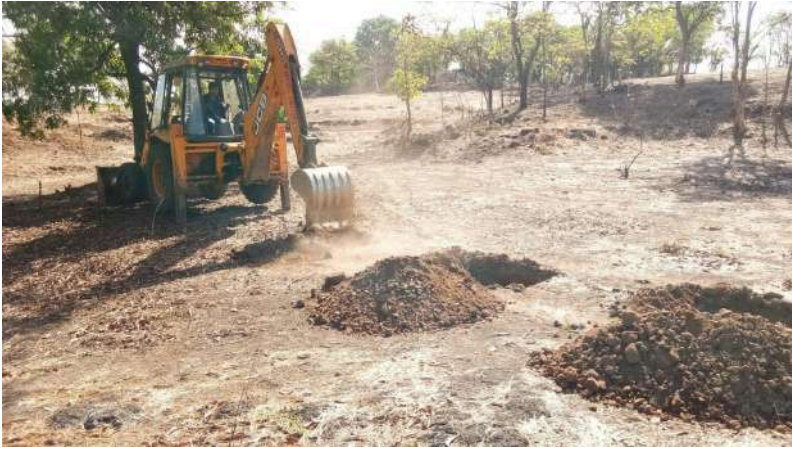
Using JCB make pits of 3 x 3 x 3 feet
